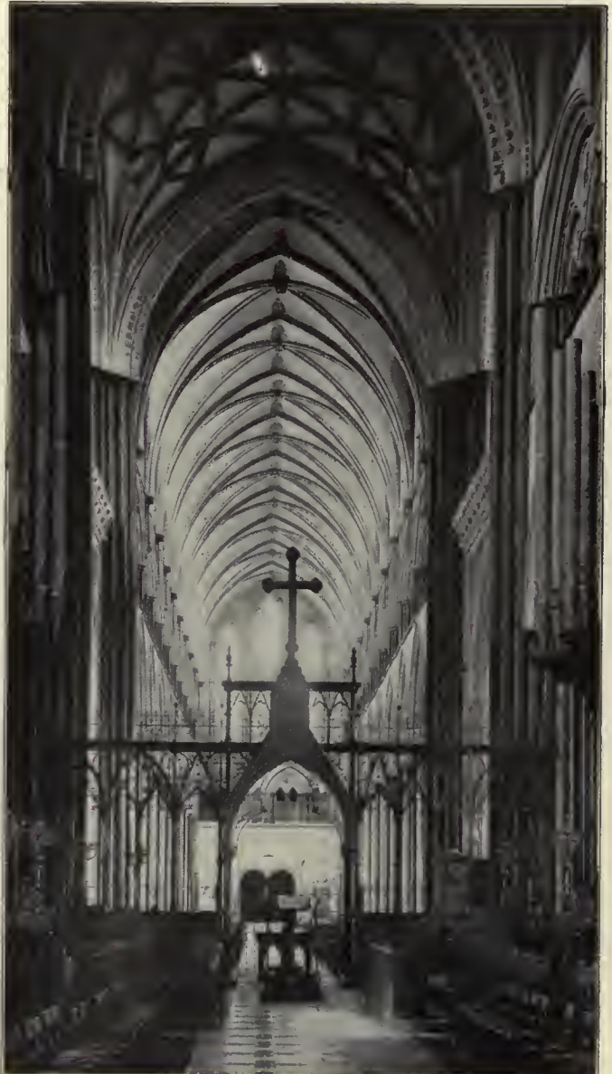
Photo, F. Frith & Co. Ltd. FIG. 16.—EARLY ENGLISH LIERNE VAULTING. Tower of Salisbury Cathedral.
